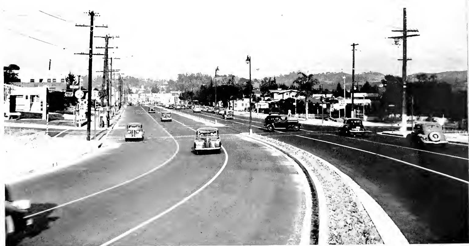
Colorado Blvd. Divided Highway in Los Angeles County paved with 2-inch asphaltic concrete on 6-inch Portland cement concrete base
